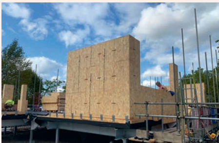
Top Knox Bhavan's riverside March House in Berkshire. Above The SIPs panels saved programme time and dealt well with challenging site logistics. Above right The simple insulated timber panel construction methodology.
