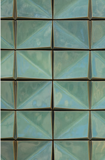
Above Detail of the locally-sourced 3D Darwen terracotta green faience tiles that were especially created for the project.
