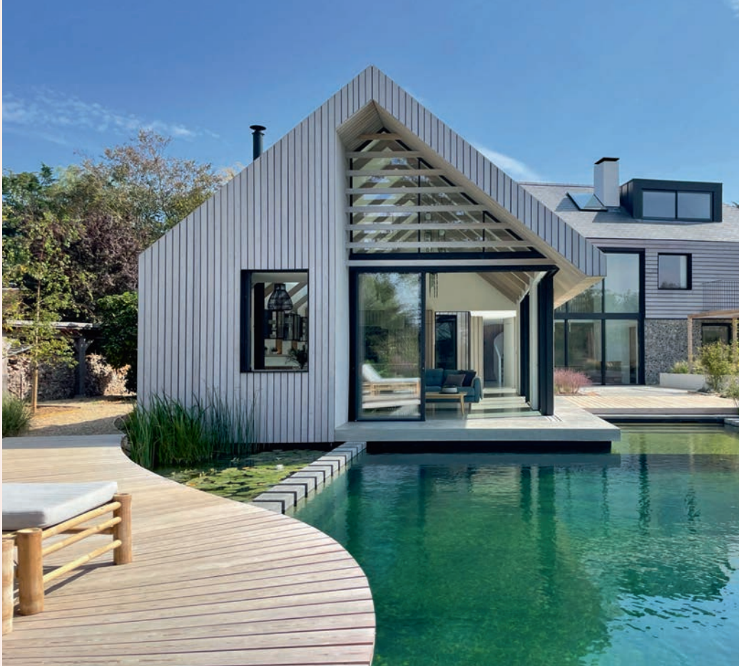
Above Siberian Larch cladding used to create a beautiful waterside retreat. Images courtesy of Studio-Fuse.
