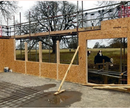
Above View from the mezzanine showing the use of wooden furniture to complement the OSB. Left The SIPs exposed in the external lobby before being covered with white metal cladding. Below SIPs enabled assembly of the office shell within a week.
