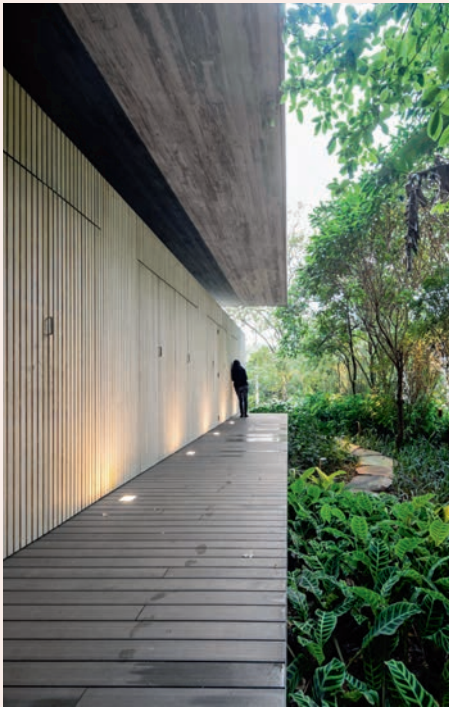
Below Accoya cladding installed vertically to create a modern look.
