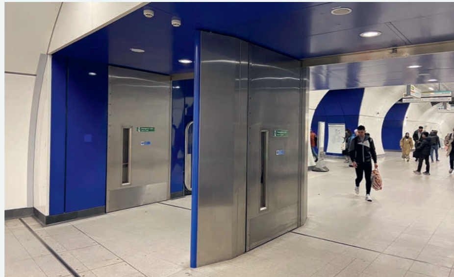
Above Bank Station, London – Double Leaf Fire Doors. Far left Insulated door (RHS) versus uninsulated fire door. Left Fire door test – 4.32m wide x 2.8m high.
