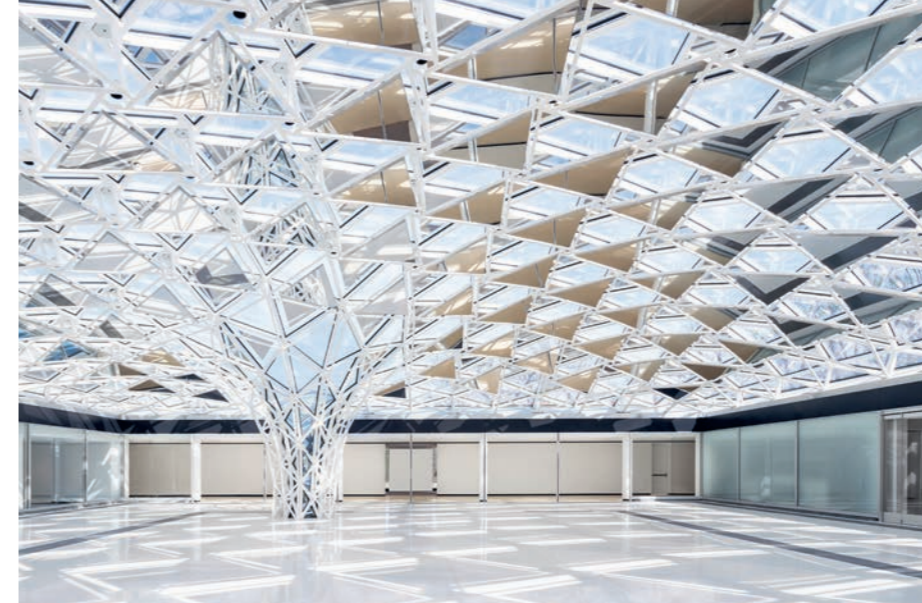
Left Common Sky's faceted mirrored inner surface creates kaleidoscopic visual effects for the museum's visitors. Below The clever double skin structure allows the structure to have a very low arch.
