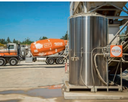
Right CarbonCure technologies enable concrete producers to add captured carbon dioxide to the production process, converting it into a mineral and reducing the carbon footprint.
