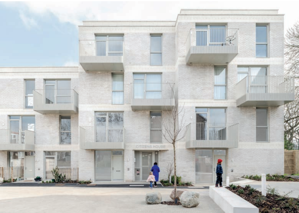
Below Big bolt-on balconies bring a real punch to the principal facade, creating greater depth for the staggered block form.
