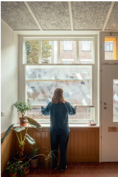
Above A secondary internal sash, fitted with obscured glass, allows privacy or visibility to the street.
