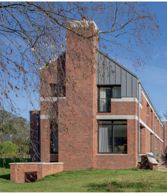
This image The main residential wing overlooking the courtyard: materials palette of brick in two colours, pale stone and zinc. Left The two-storey wing terminates in the chimney for the ground-floor living room.
