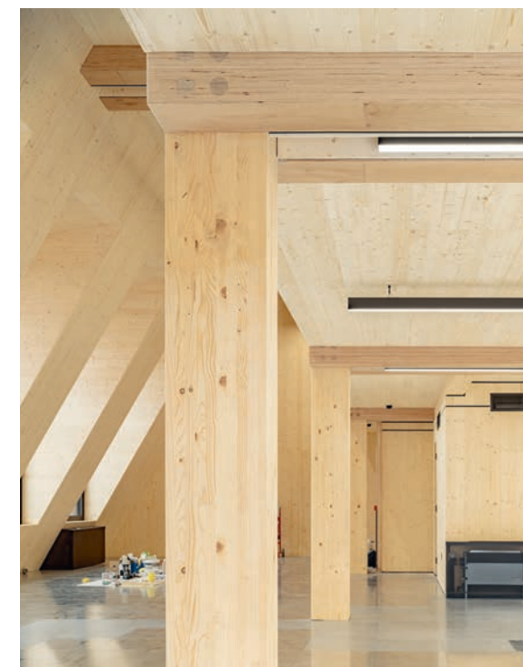
Above An arched window was incorporated into the upwards extension, echoing a feature of a past building on the site. Left An extension of glulam beams and CLT floors, walls and roof provides highly insulated, additional office space.
